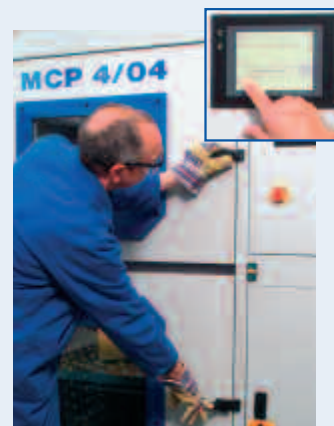
Close the doors and let the PLC controller take over.
