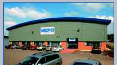
Head-Quarters, Demo, Development and Manufacturing Facility, Stone · England
